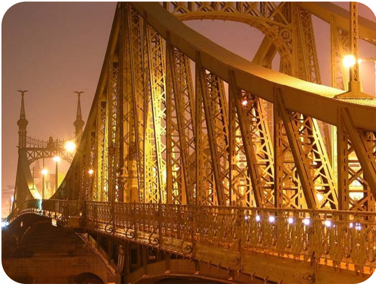
The Freedom Bridge in Budapest.
